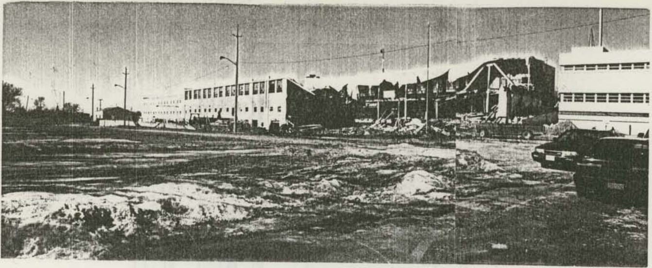
"Coming down" Front of building 14
